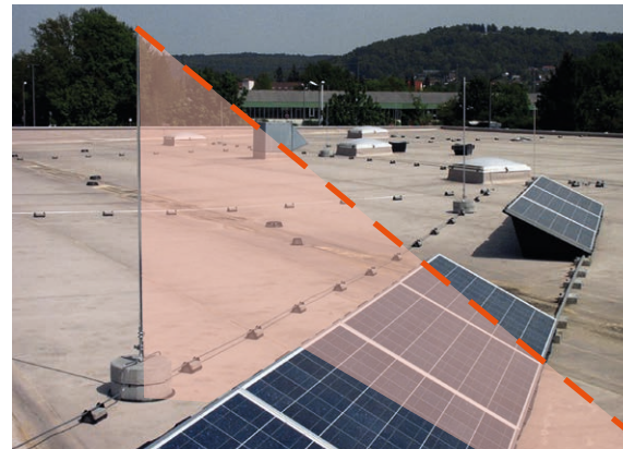
Figure 12 Determination of the protected volume using the protective angle method
