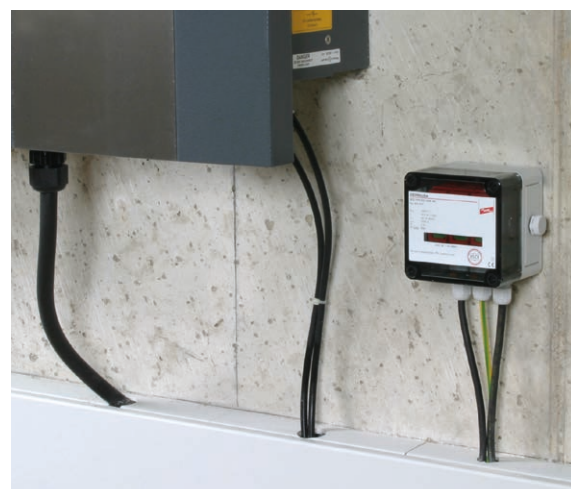
Figure 14 DEHNgard M YPV SCI 1000 1M type 2 arrester for protecting inverters (1 MPPT)
